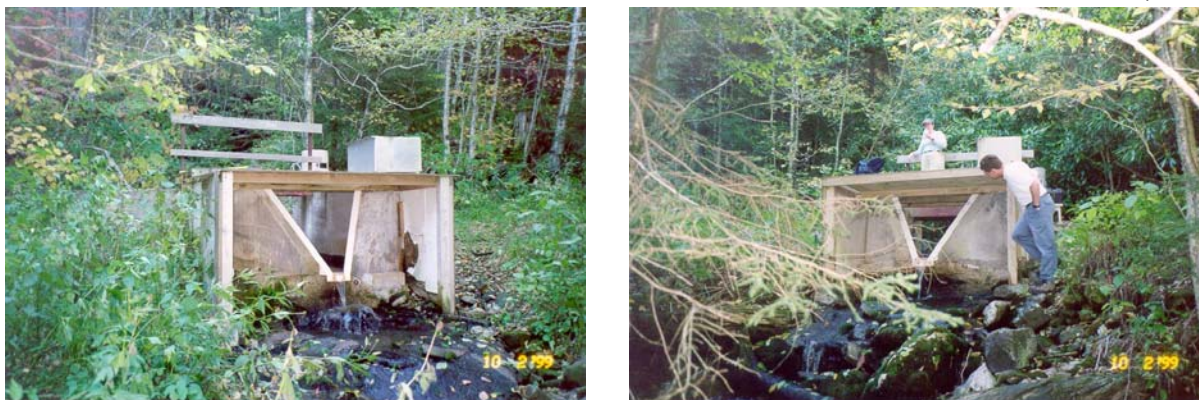
Figure 3.1. Southwest and northeast weir stream gages, respectively.
