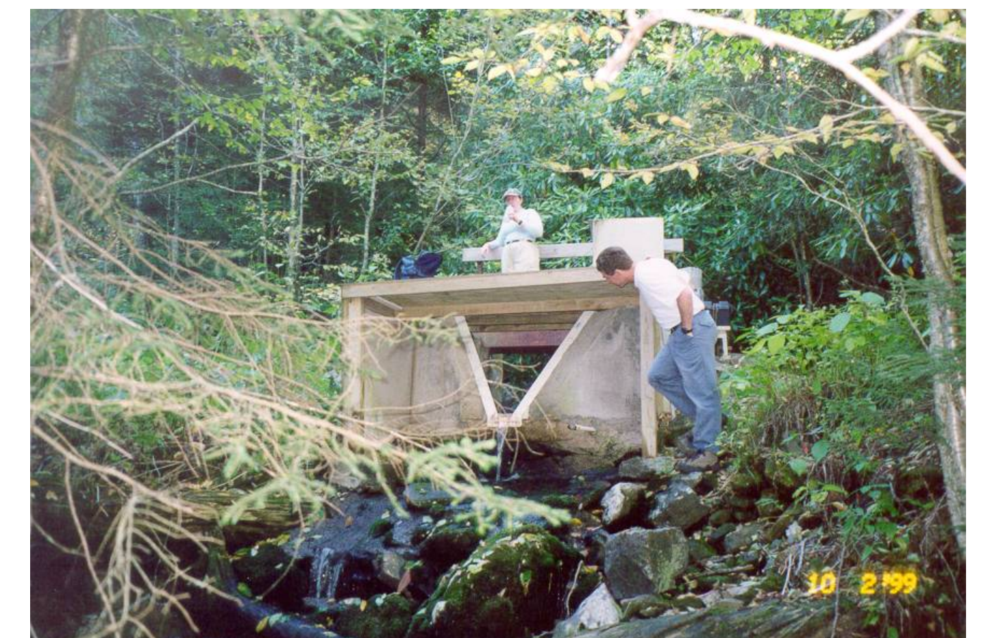
NDW Stream Gages, SW and NE Weirs, respectively.
