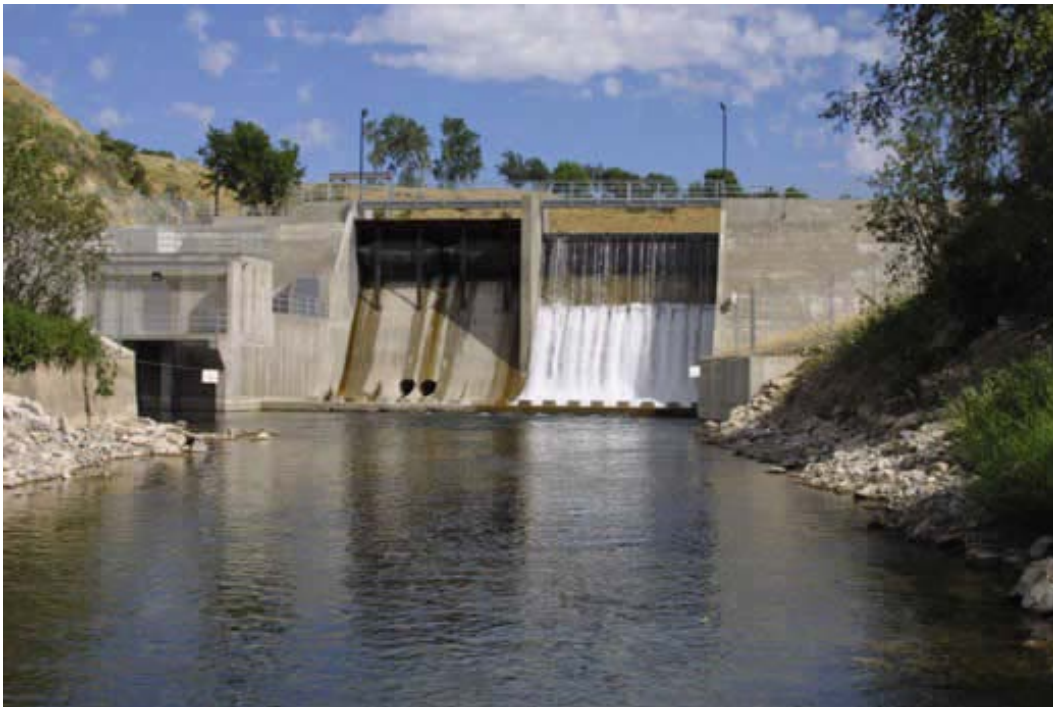
First Dam after 2002 Rehabilitation (Summer 2002)
