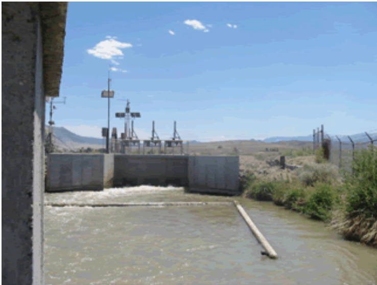
Figure 1. An Automated Gage on the Sevier Valley/ Piute Canal
