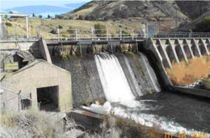
Logan First Dam is a small concrete dam and powerhouse.
