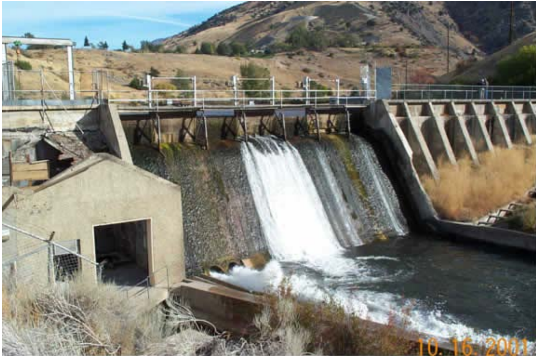
First Dam prior to 2002 rehabilitation (Fall 2001)
