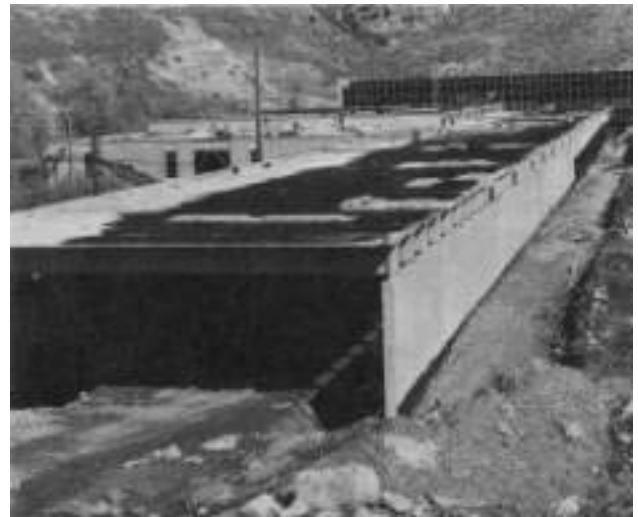
Rearview of laboratory during construction
