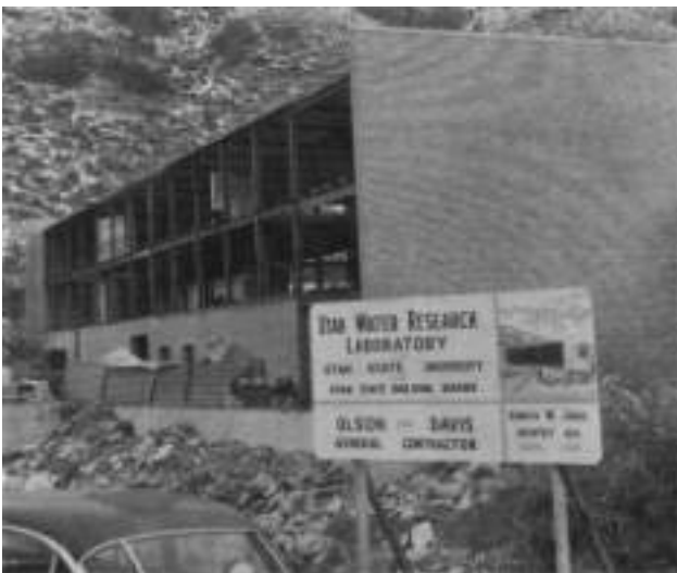
Front view of laboratory as construction progresses
