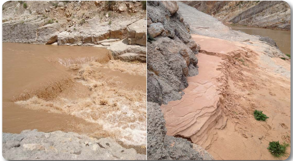
The Virgin River Gorge fish barrier during a flood event and sedimentation near the fish barrier following a flood event
