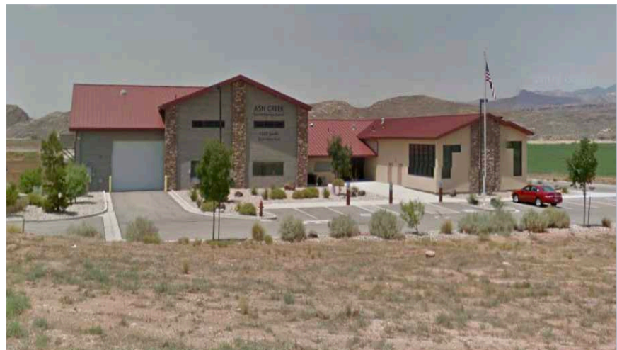
Figure 1: The new demonstration site will be located at the Ash Creek Special Service District in Hurricane, Utah.
