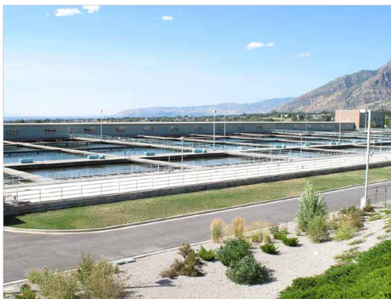
Figure 1: Little Cottonwood treatment plant ponds.
