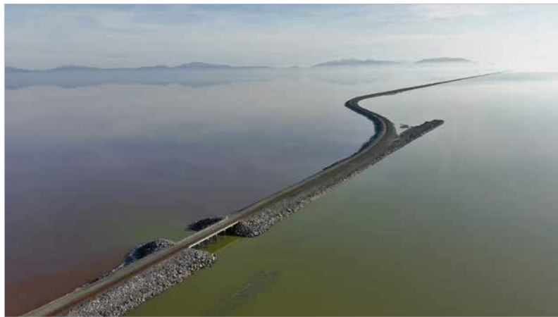
Figure 1: The Great Salt Lake's West Crack Breach
