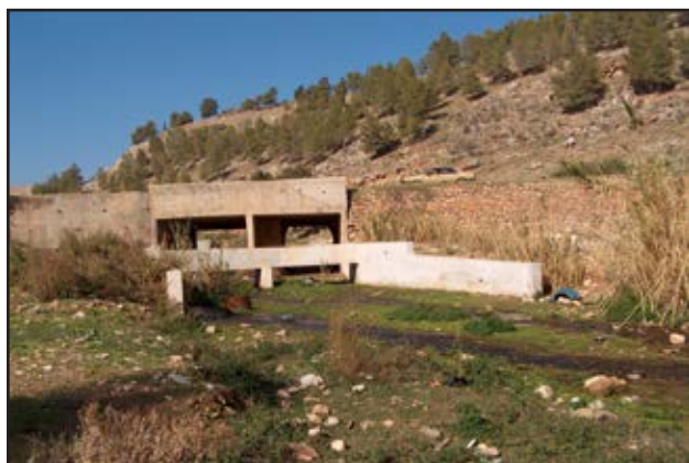
A flow measurement flume and bridge on a tributary to Wadi Fara (Occupied Palestinian Territories)
