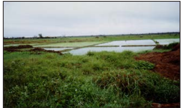
The results of investments in irrigation facilities that integrate modern and ancient structures: The first crop of rice grown in the Madroya region in nearly 1,000 years (Mahaweli River Basin, Sri Lanka)
