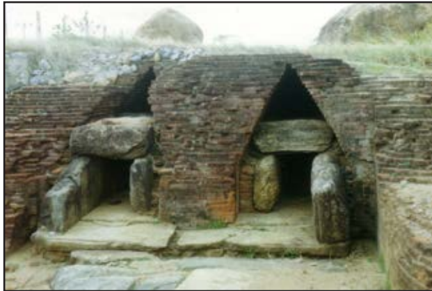
Two-thousand-year-old outlet works from a dam on the Madroya River in Sri Lanka. These ancient structures and the large dam from which they drew their water were in the same location as a modern dam and outlet works designed to serve the same irrigated area (Mahaweli River Basin, Sri Lanka)
