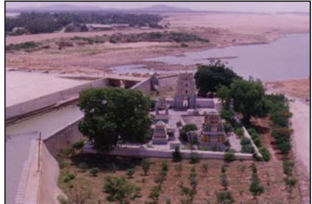
Stilling basin and an ancient Hindu temple downstream of a major dam on the Pennar River (Andhra Pradesh, India)
