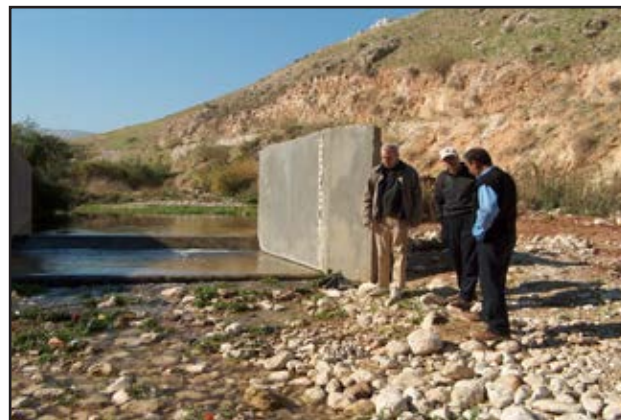
Inspecting a flume for measuring and recording flows in the Wadi Fara Watershed near Nablus, West Bank (Occupied Palestinian Territories)
