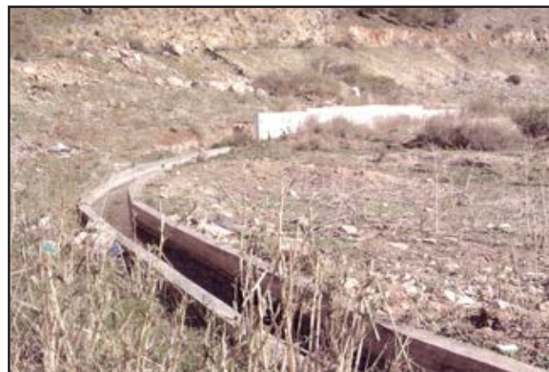
An irrigation canal (approximately 0.5-meter in width) which diverts water from Wadi Fara to Palestinian farmers in the valley (Occupied Palestinian Territories)
