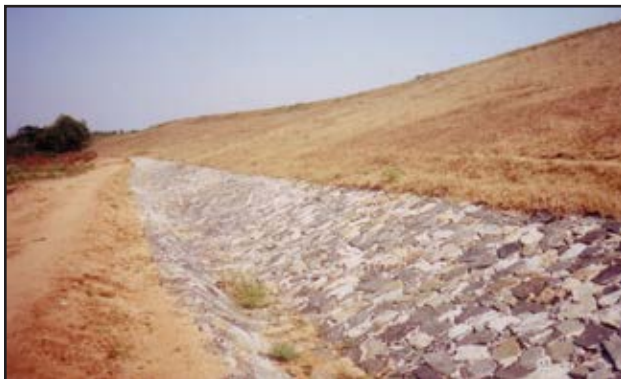
Modernized toe-drain on an ancient "tank" (Mahaweli River Basin, Sri Lanka)
