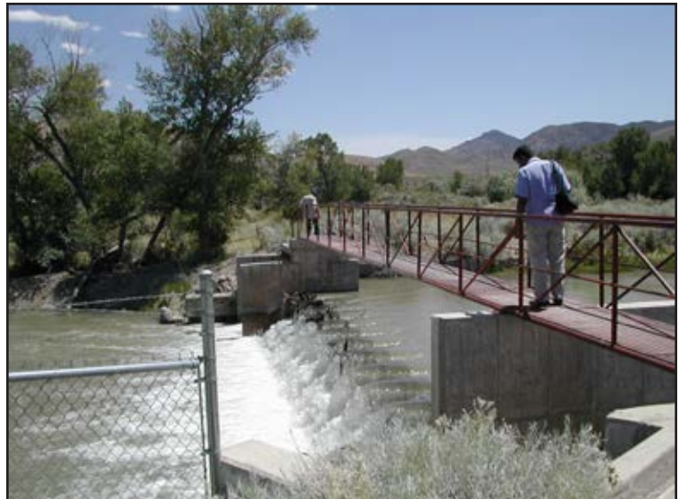
Diversion structure for the Richfield Canal in the Sevier River, Utah
