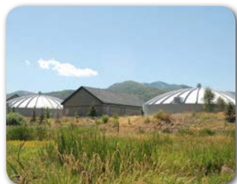
Wastewater Treatment Plant at Snyderville, Utah
