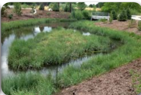
Stormwater wetland treatment channels can retain the contaminated water to allow for decomposition and uptake of pollutants by wetland plants before the water enters the river
