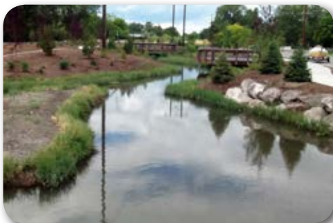
Stormwater wetland treatment channels can retain the contaminated water to allow for decomposition and uptake of pollutants by wetland plants before the water enters the river
