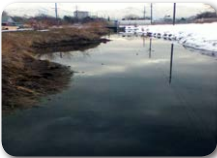
9th South stormwater channel to be upgraded to a treatment wetland
